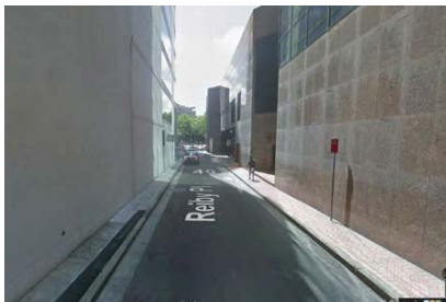
Existing condition - Reiby Place
